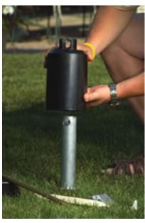
4. Drop plastic sleeves over installed Aussie Augers.
