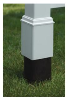
6. Slide assembled arbor side panels over plastic sleeves.
