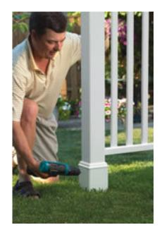
7. Install fastening screw through the base molding to secure the arbor to the plastic sleeve.
