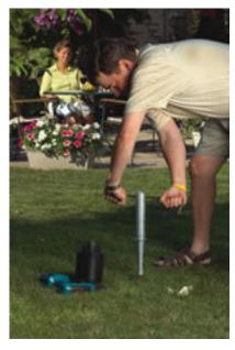
3. Screw the Aussie Augers into the ground. Apply water before starting in extremely dry conditions.
