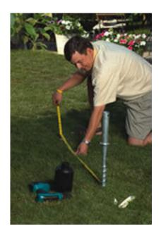
1. Identify the "footprint" of the arbor and move temporarily. Ensure that the location of the Aussie Auger Anchors are square
